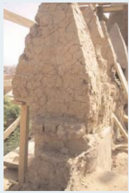
(Left) The exposed parapet pillars following removal of the cement. (Right) the northeast corner of the mosque during the removal process.
