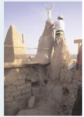
(Left) The exposed parapet pillars following removal of the cement. (Right) the northeast corner of the mosque during the removal process.
