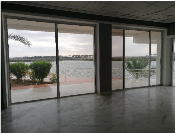
Figure 32 View facing south (plaza and river)
