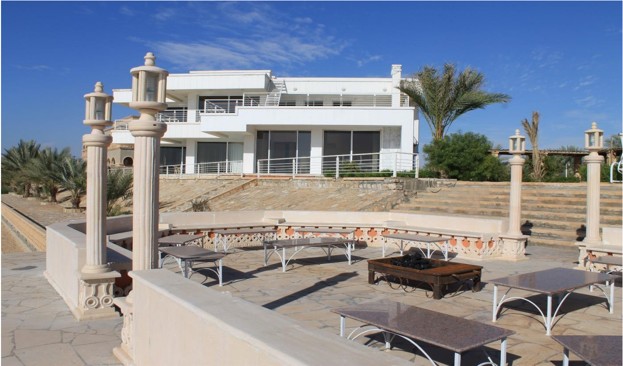
Figure 55 View from midlevel Msanayeh to the upper plaza and the house
