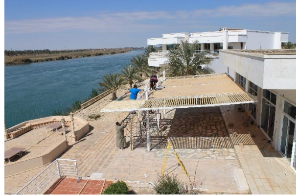
Figure 64 Canopy under construction
