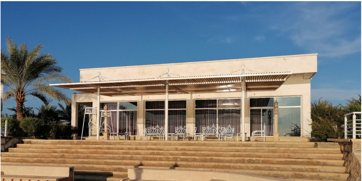
Figure 46 Dewan western façade overlooking the Euphrates river with deep canopy protecting the glass facade
