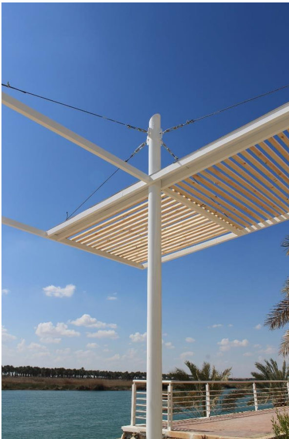
Figure 65 Light weight steel structure
